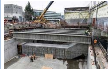
Girders over north SR99 tunnel 01.04.18
