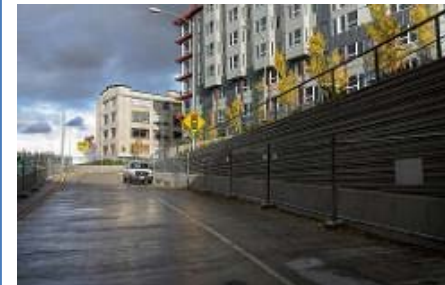
NB SR99 off-ramp to Dexter Ave 11.15.17
