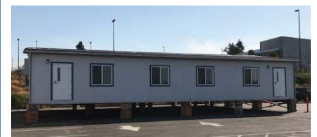
Replacement Field Office
