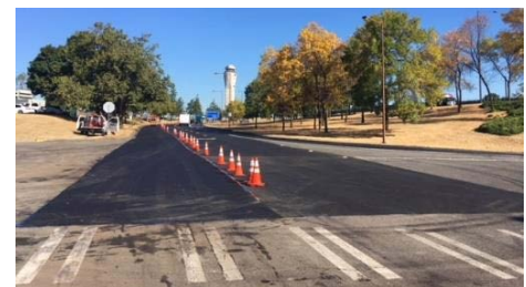
Air Cargo Rd Pavement Repair
